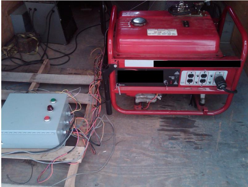
**Figure 2.3:** Modular EMS equipped generator. Modules housed in grey electrical box and connected to generator hardware via custom wiring harness.
